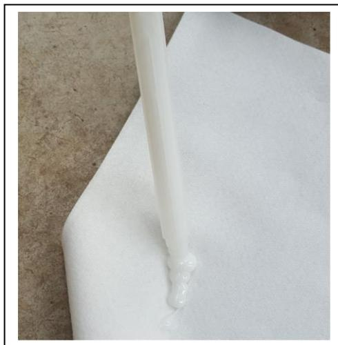
**Step 5.** Apply the epoxy. I ran the epoxy in 3 lines on the bottom half of the headstone. This resembles the conditions in a cemetery where the top is broken off and the bottom is stuck in the ground yet. I should have applied the epoxy to the top and bottom breaks but in the excitement I forgot to do it. I must have used the right amount by the way it worked.
