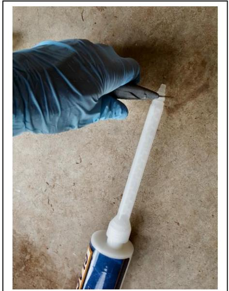
**Step 4.** Squeeze 2 inches out before using the product. You do not want to apply epoxy that hasn't mixed. It will not set up. The nozzle is designed to mix the epoxy by the time it is out but this assures that it is mixed for use. The tube is designed with 2 compartments and the product is pushed out evenly from both compartments.
