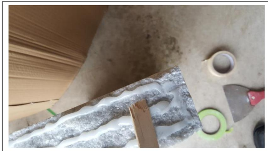
**Step 7.** Set the top in place. You should try and wiggle the top in place but when I set the top on, it stayed right there. No movement. It is hard to see on the photo but the product squeezed out but this gave me the idea that I used enough product. This is better than not having used enough epoxy.
