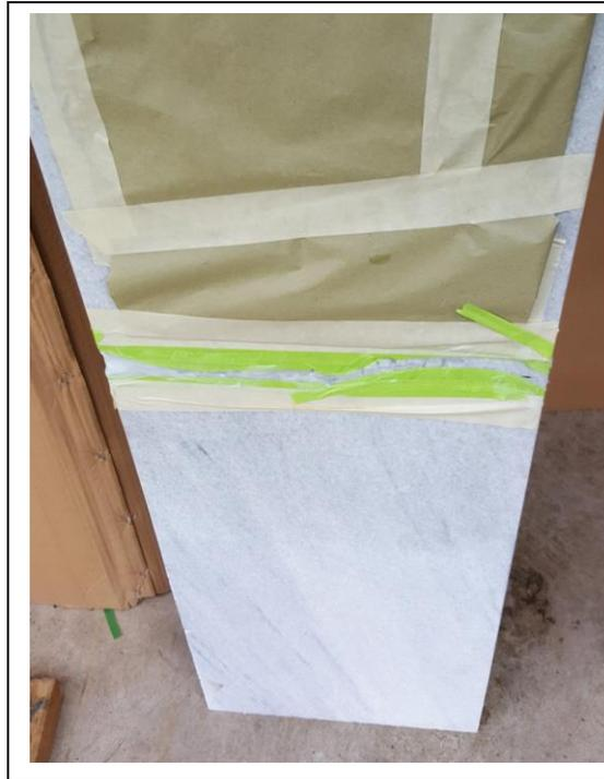
**Step 8.** Wait about 10 minutes and remove the tape around the break while waiting. Pull the tape away from the seam area. When the excess epoxy feels like rubber you need to trim the excess from the stone. I used a razor blade set sideways in a handle and scraped along the stone flats. It gave a clean finish to the seam.
