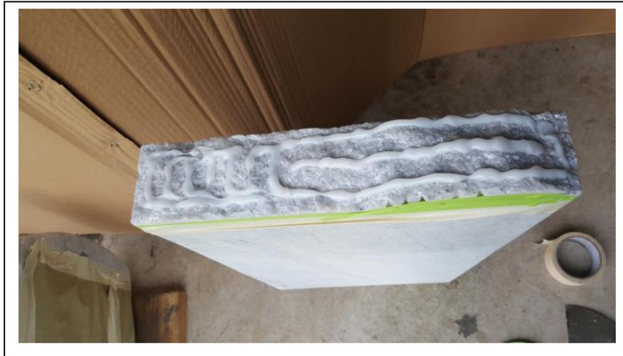
**Step 6.** Spread the epoxy evenly. I used part of a paint stick to spread the epoxy as even as possible covering the whole face of the broken area.
